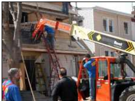
Crews were hard at work, halfway through on Thursday afternoon. Winston Peter's home had been partially destroyed by a fire. (Christopher Henderson)
